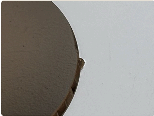
The bite left by a starter hole drilled flush with the line.
